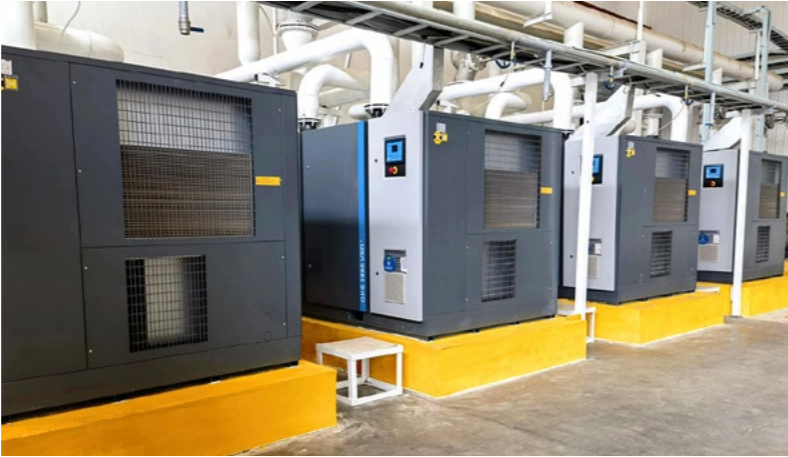
Water Ring Pump Renovation Equipment of Xianning Plant
