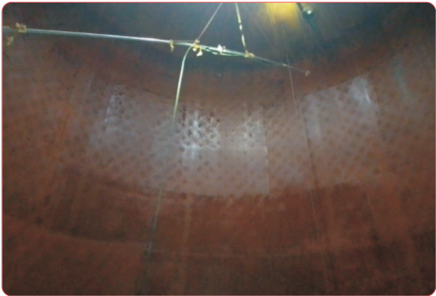
Intelligent high-pressure tank cleaning operation
