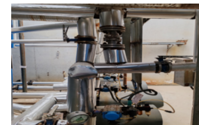
Addition of Concentrated Water Pipelines for Desulfurization and Denitrification
