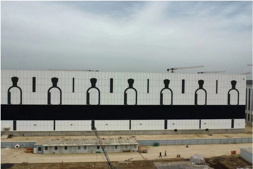
Facade Photovoltaic Project at the Intelligent Industrial Park of Gujing Distillery
