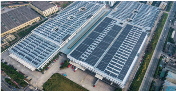
Solar photovoltaic arrays deployed in the factory area
