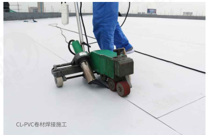
CL-PVC卷材焊接施工
