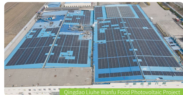
Qingdao Liuhe Wanfu Food Photovoltaic Project
