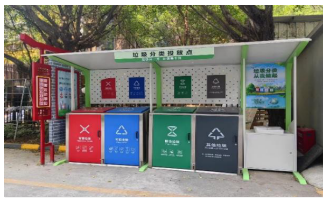
Waste Sorting Area
