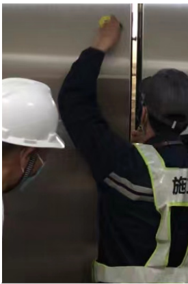
Engineers opening the elevator door
