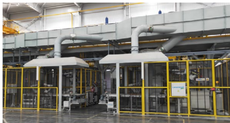
封闭式设备+负压抽排 The Enclosed Equipment and Negative Pressure Extraction
