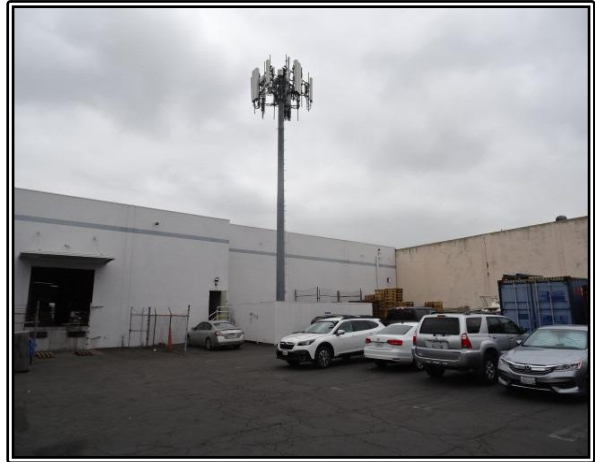
Cell tower on southeasterly side of subject lot.
