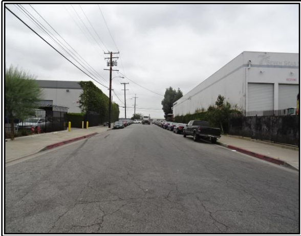
Northwest view of Date Street.
