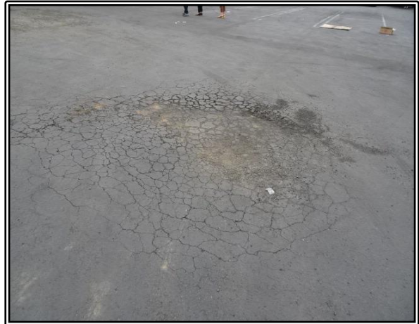
Portions of the asphalt paving are in fair condition.
