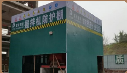
封闭式搅拌机防护棚
