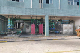
Closed-Loop Water System with Plate Heat Exchanger
