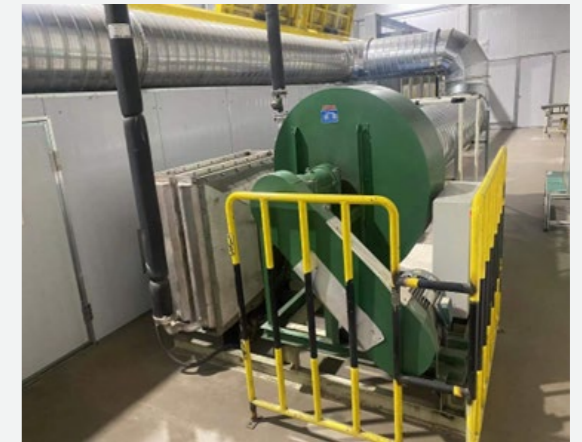
Heat Recovery Retrofit for Air Compressors
