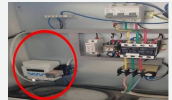
Electrical Upgrades on Workshop Doors
