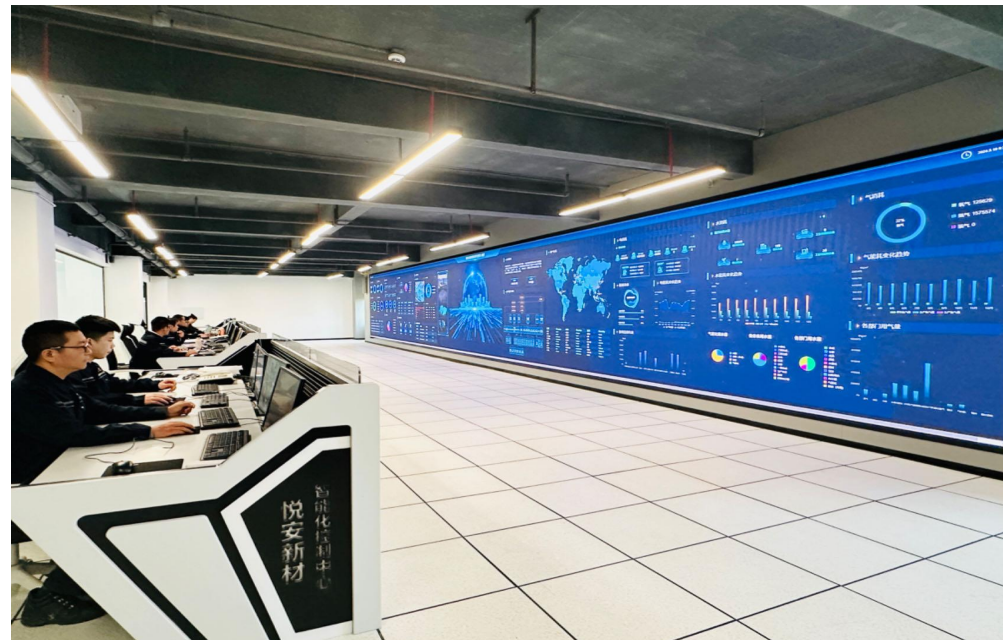
YueAn Smart Control Center
