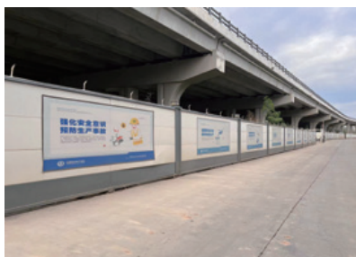
▶ 施工围挡及外架100%全封闭
