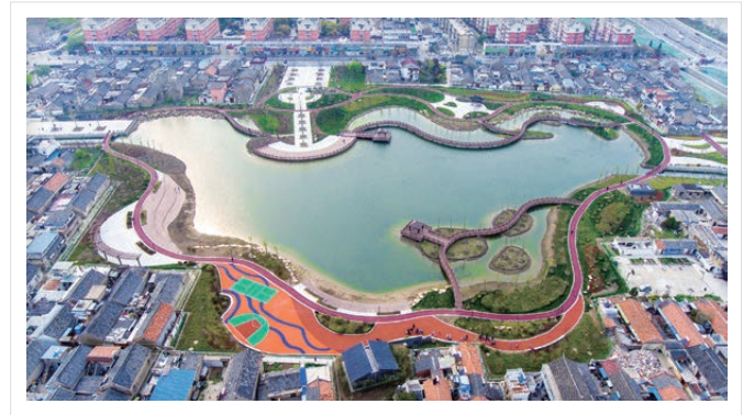
整治后的淮安黑臭水体综合整治项目 Comprehensive improvement project of Huai'an black and odorous water after improvement
