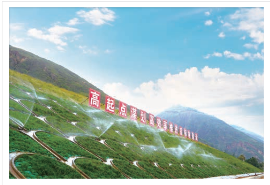
边坡绿化自动喷淋系统 An automatic spraying system for side slope greening
