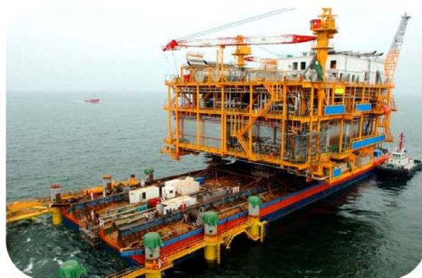
“浮托法”安装旅大项目万吨级组块
